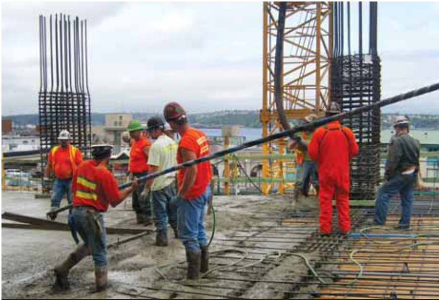
Ironworkers on a downtown Seattle condo get ready for another pour.
