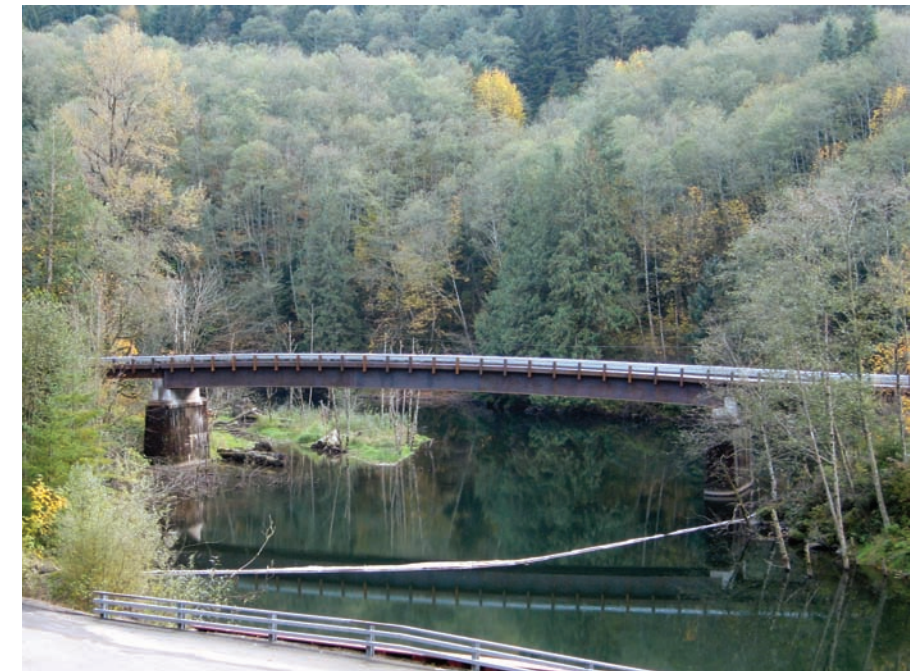
One Mile Bridge Replacement
